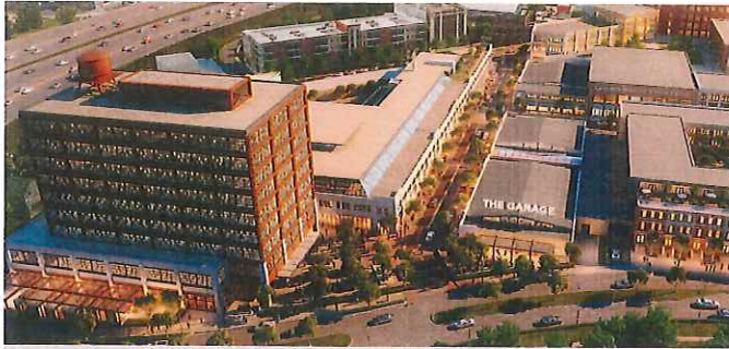
Hendricks Commercial Properties is transforming the old Coca-Cola bottling plant in Indianapolis into a $260 million mixed-use development, featuring 180,000 square feet of office space, a boutique hotel and food hall.
