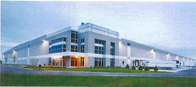
RGLP Intermodal North 9224 is a 482,220-square-foot bulk warehouse within Duke Realty's Rickenbacker Global Logistics Park in Columbus, Ohio.
